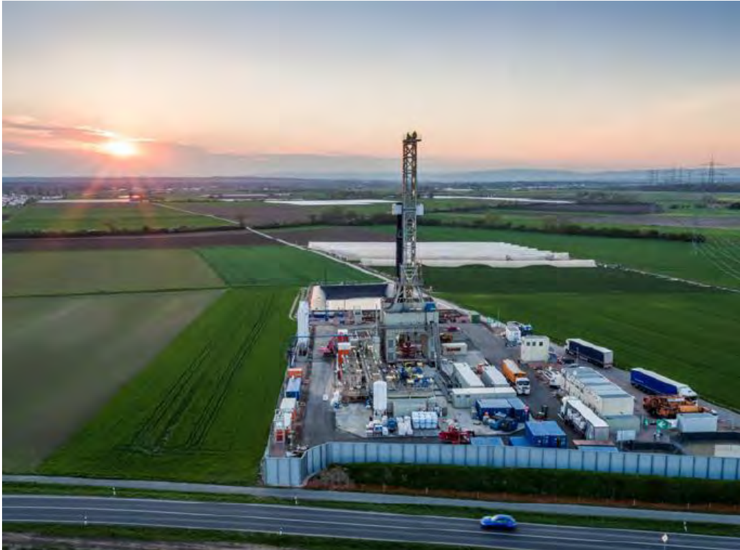
Obr. 45 - Vrtná souprava MND Bentec 450 (MND Drilling & Services a.s.)
